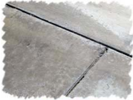
A CLOSE LOOK AT SOME DRIED CONCRETE FROM A SIDEWALK.
